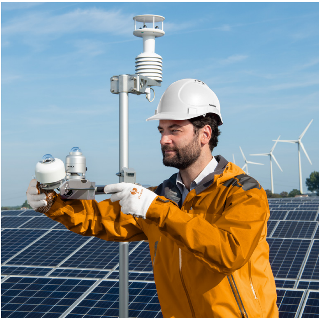
Figure 2 Two SR300-D1 pyranometers—one tilted for Plane of Array (POA) measurement (left) and another mounted horizontally for Global Horizontal Irradiance (GHI) measurement (right).
